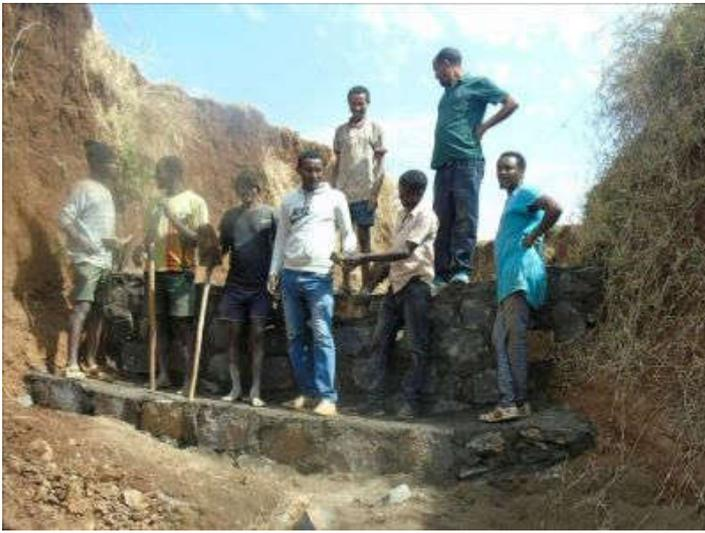
**Bees for Development Ethiopia** is recovering degraded land in the **Lake Tana** catchment area. This image shows one of the stone arc weirs we have built to stem the erosion in this active gully in **Yisala**. We are working to reverse land degradation and to **restore bee habitat and safeguard the livelihoods of Lake Tana beekeepers**.
